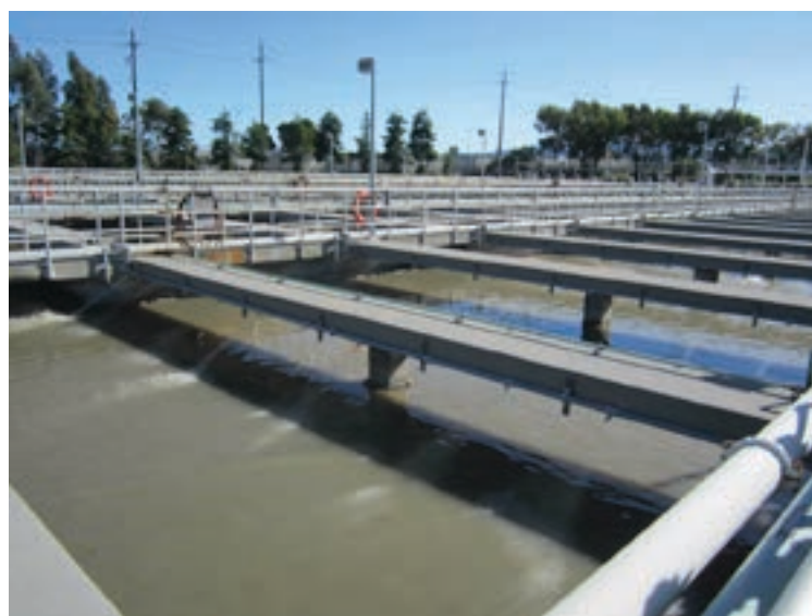
Primary Sedimentation process
